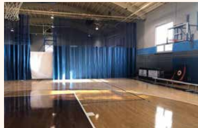
△ With help from General Mills and other sponsors, the facility was renovated with new bathrooms, windows, heating and air conditioning and electrical system, a refurbished kitchen, gymnasium, computer lab, reading lab and art rooms.
