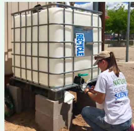
△ Donated intermediate bulk containers being installed for rain collection
